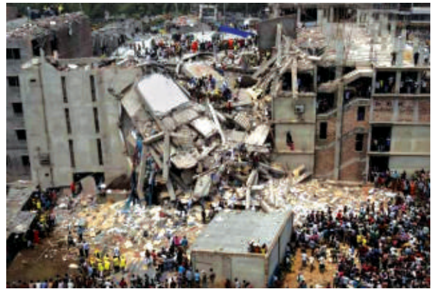
Rana plaza after collapse, Photo Credit: http://img.wikinut.com/img/3yx0v86i3it_mqyd/jpeg/0/Rana-Plaza-Collapse.jpeg
